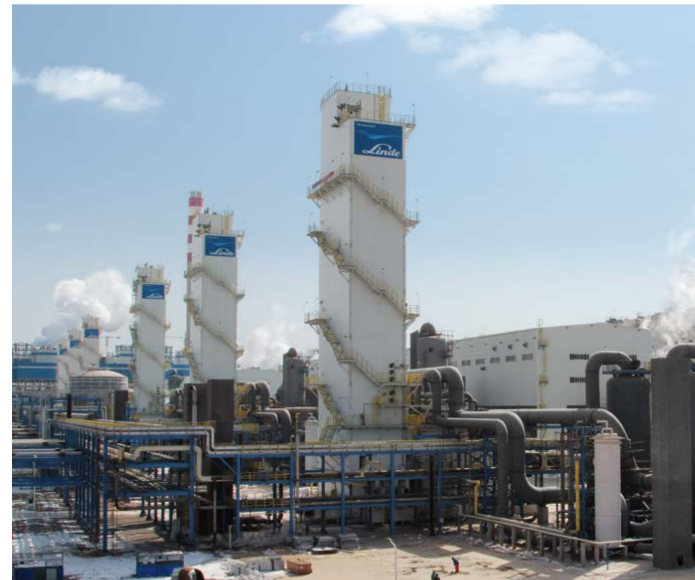
Air separation units near Yinchuan City, China.
