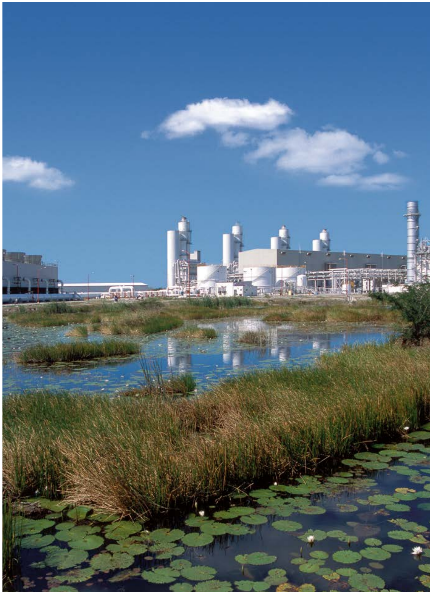
The air separation units at Cantarell (Mexico) were planned and built by Linde's Engineering Division.
