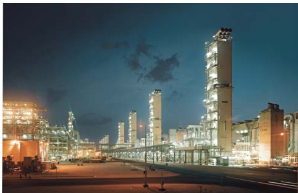
Air separation units at the Pearl GTL complex in Ras Laffan, Qatar.
