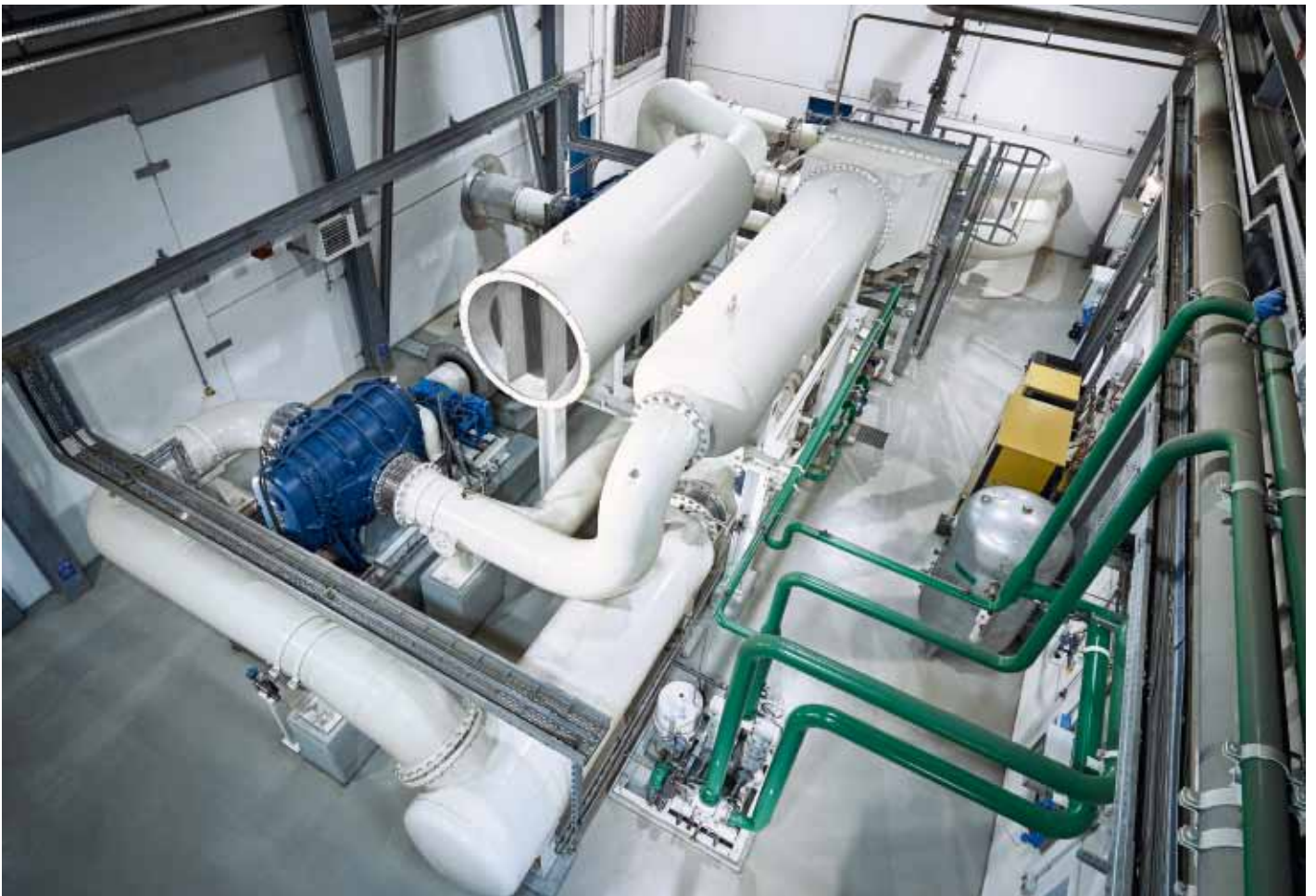
VPSA plant for 2,400 Nm 3 /h (82 tpd) oxygen product for steel plant in Italy.
