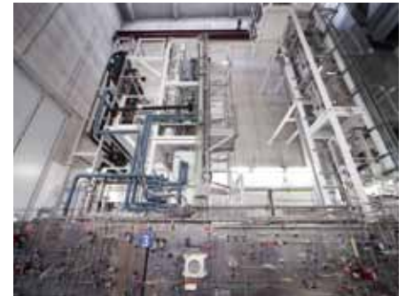
EDHOX™ demonstration plant
