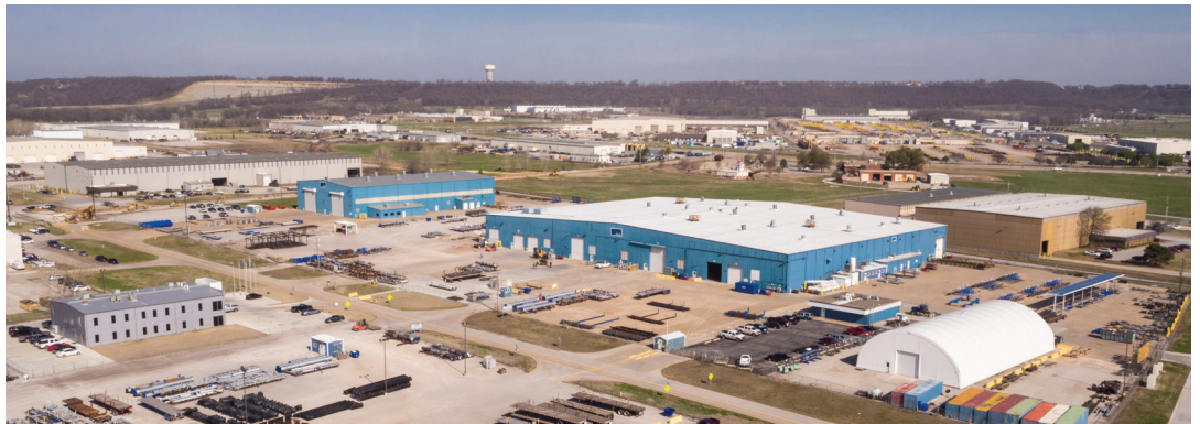
Linde fabrication facility, Catoosa, OK USA
