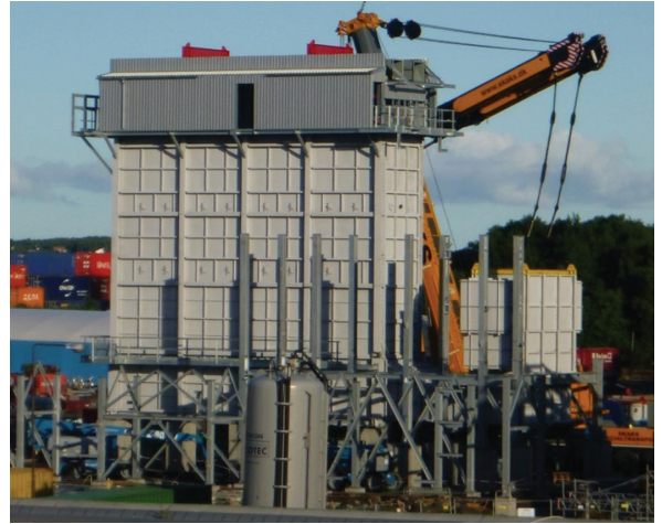
HYDROPRIME® Max under construction
