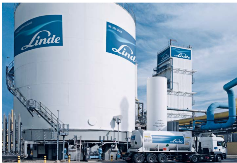
Liquid Air Energy Storage (LAES) tank at an air separation plant in Leuna, Germany.
