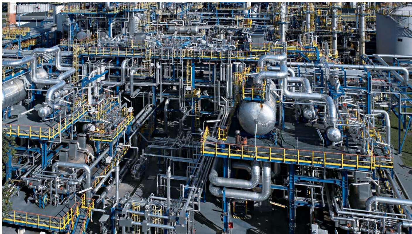
Two of the four Claus units at the Polish refinery in Gdansk that are being engineered for increased capacity through oxygen enrichment.
