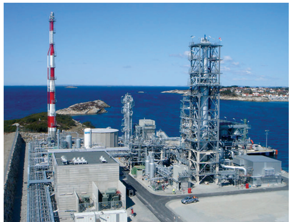
The mid-scale LNG plant above, with 900 tonnes per day net liquefaction capacity, is located in Stavanger, Norway, and uses the Linde processing technology
