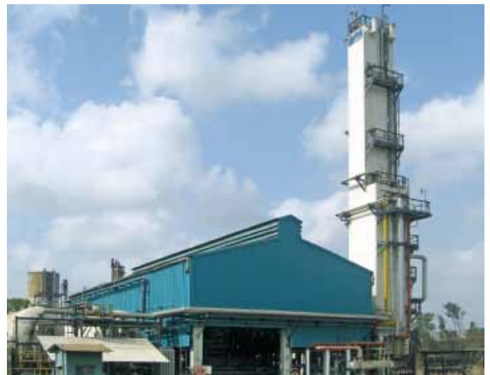
Plant for the recovery of liquid argon from ammonia synthesis purge gas in Hazira, India.
