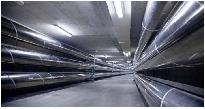
Gas-insulated high-voltage transmission line in tunnel. Reference: Siemens Erlangen, 380 KV GIL for the Paulaner brewery in Langwied, Munich.
