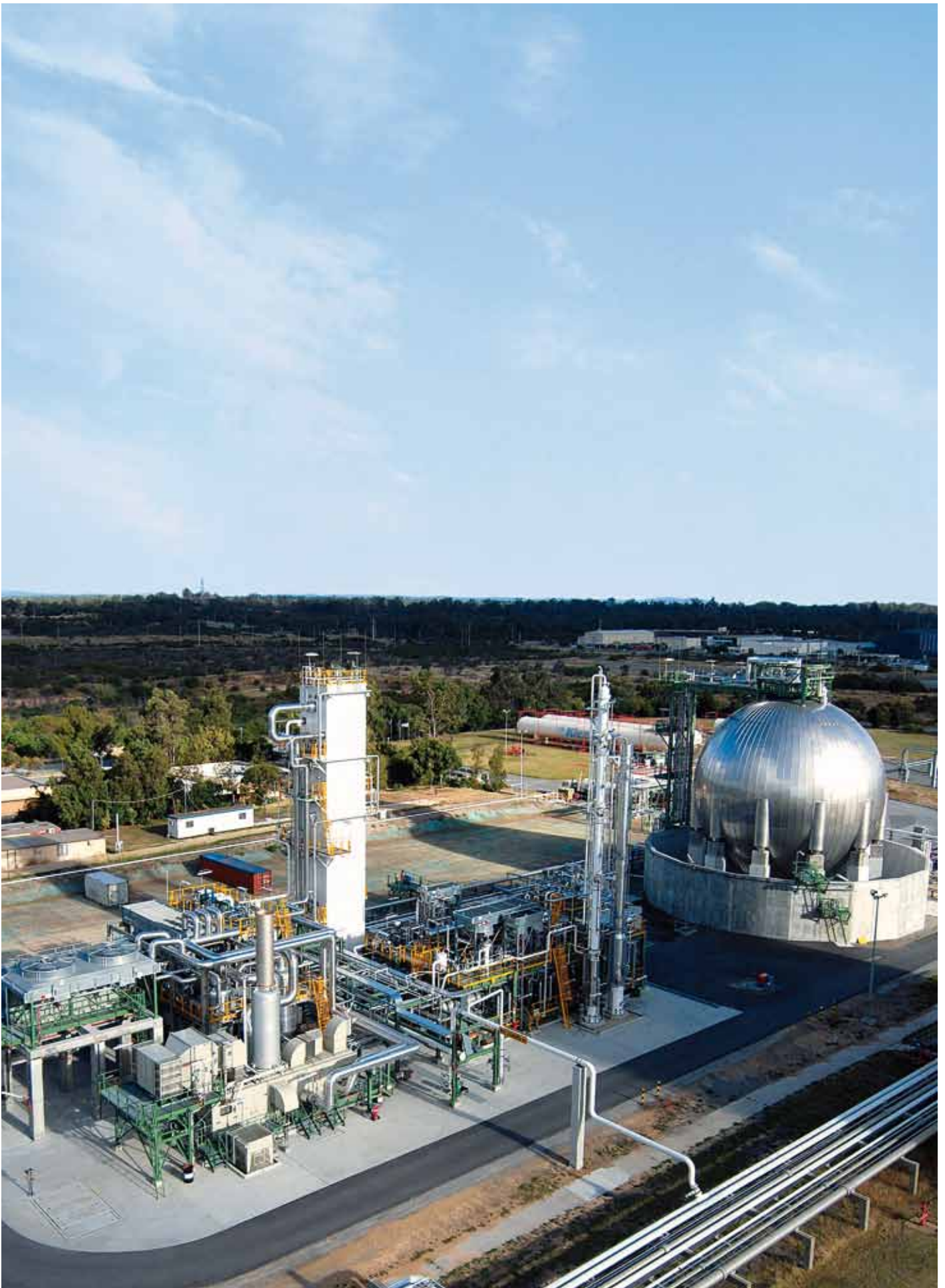
Small-scale StarLNG® plant with 175 tpd liquefaction capacity in Kwinana, Australia.
