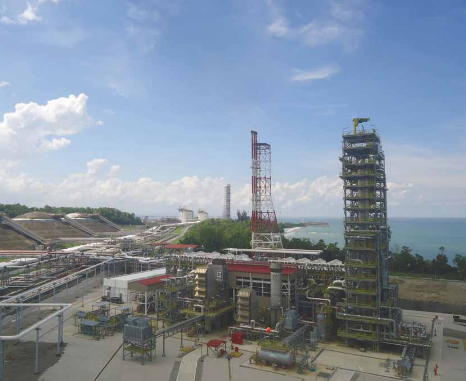
Mid-scale LNG plant with up to 0.8 mtpa liquefaction capacity located in Bintulu, Malaysia, on stream since 2015 and featuring Linde's LIMUM® closed mixed refrigerant cycle process with coil-wound heat exchanger.
