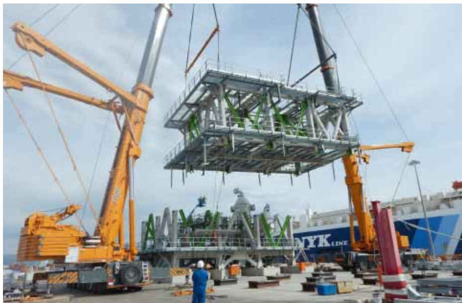
NRU module fabrication at Tarragona, Spain.
