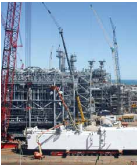
Erection of NRU coldbox at Karratha, Australia.
