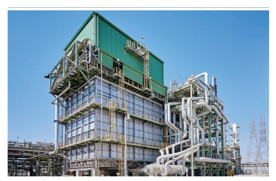
Many processes throughout the refining, petrochemical, synthesis gas and ammonia/fertilizer industries are based on the use of hydrogen produced by the reforming process, where a hydrocarbon-steam mixture is converted into a hydrogen rich gas in the presence of a catalyst at elevated temperatures and pressures.
