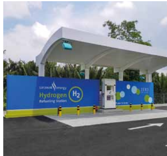
Refueling station in Sarawak (Malaysia)
